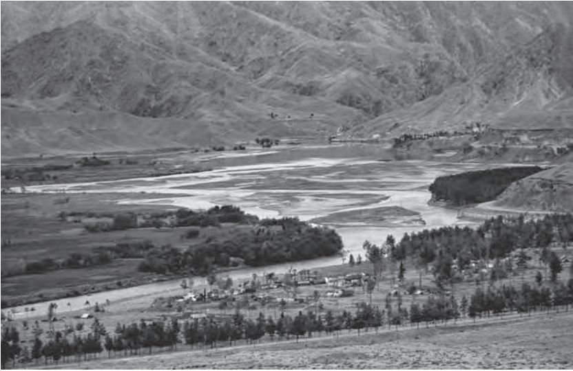
The Kabul river and the Kabul–Jalalabad highway looking downstream to Sarobi. This road was badly cut up during the Soviet era but is now repaired and resealed.
